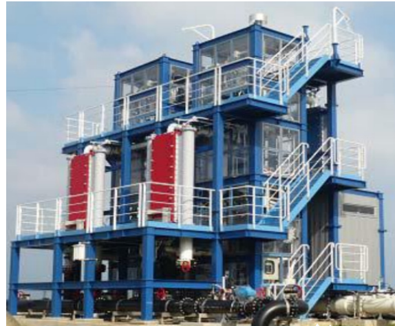
Figure 12. 50 kW OTEC demonstration power station in Okinawa, Japan. Adapted from ref. [79].
