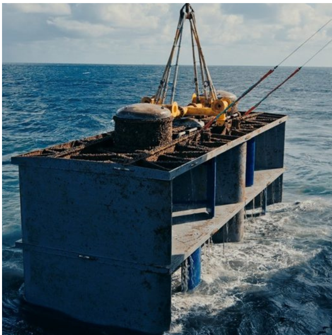
Hydroquest turbine being recovered at Paimpol-Bréhat tidal test site
