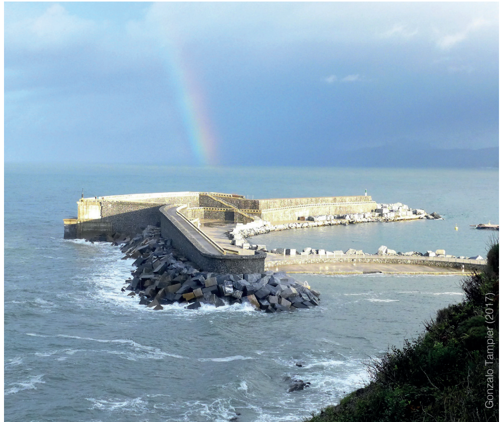
Integration of coastal protection infrastructure with oscillating water column wave energy converter in Mutriku, Basque Country, Spain.
