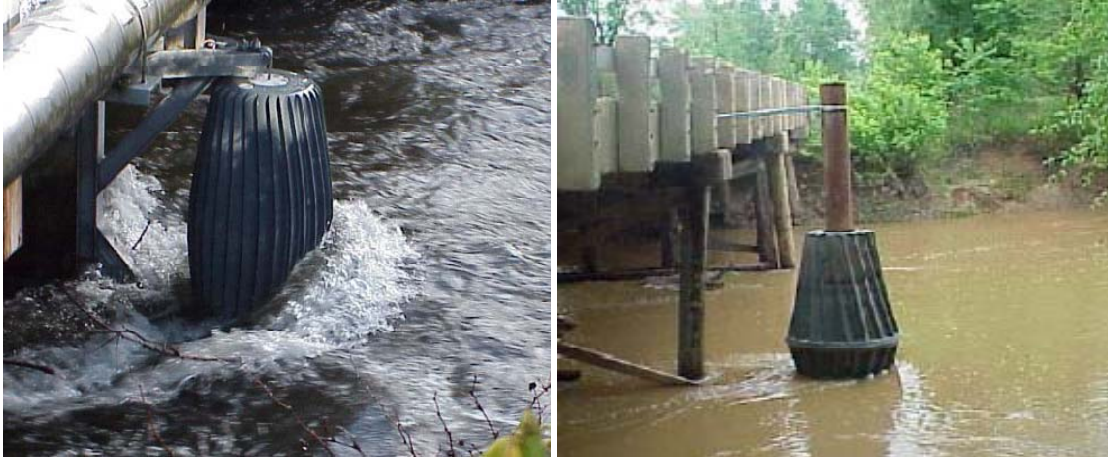
Figure 6: Debris sweepers attached directly to a bridge pier (left) and pole mounted (right) (Lagasse et al., 2010)
