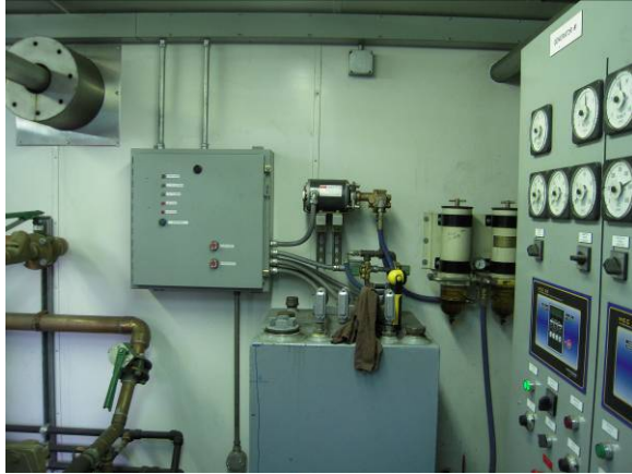
Power Plant Day Tank and Controls
