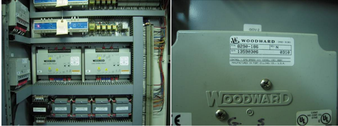
Gen-Set Controls with Load Share
