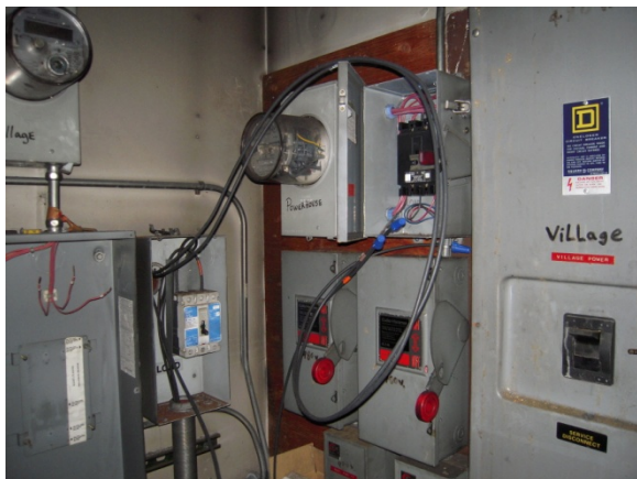
Old Power Plant – Village feeder and metering
