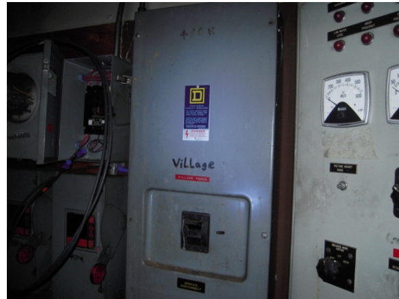
Old Power Plant – Village Feeder Switch
