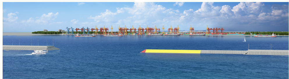
Figure 1. Bird view of a DULOW device integrated into an attached breakwater.
