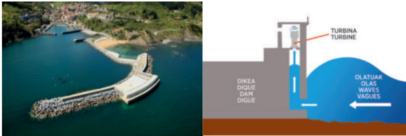
Figure 2: OWC working scheme (left) and Mutriku's power plant (right).
