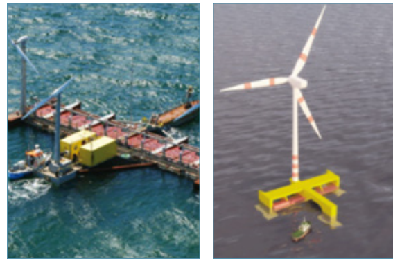
Floating Power Plant
