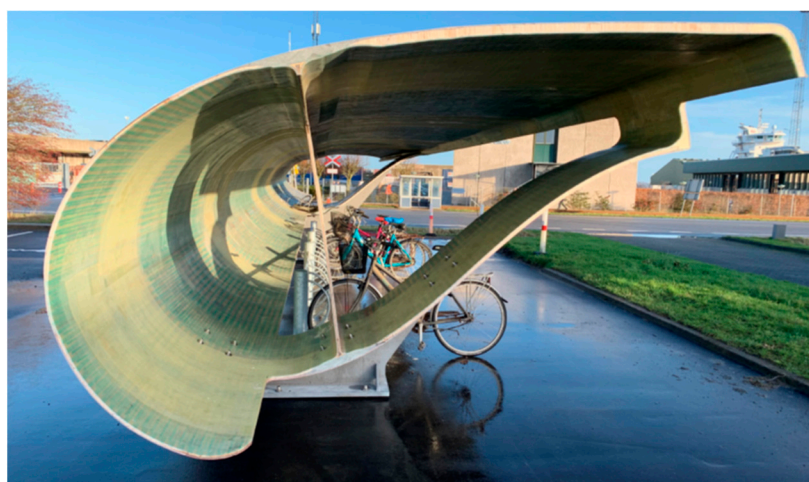
Figure 16. A reused wind turbine blade—bike shed in Aalborg, Denmark. Reproduced with permission from Port of Aalborg [177].
