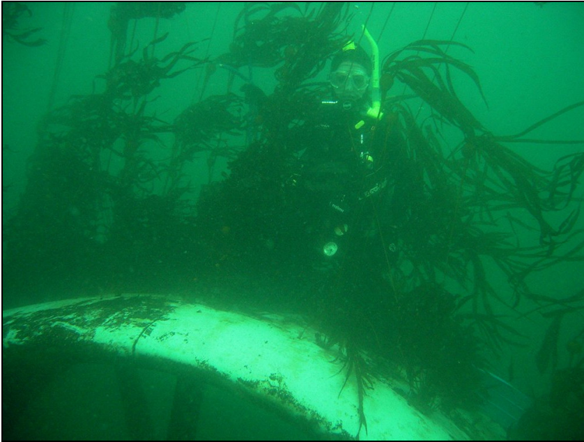
Figure 54: Algae Growing on Clean Currents Turbine
