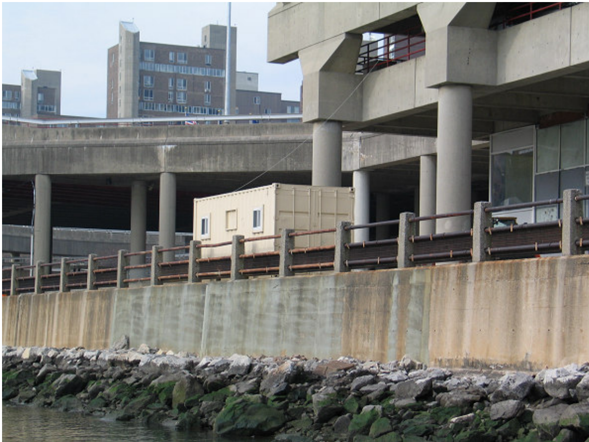
Figure 79. RITE Control Room
