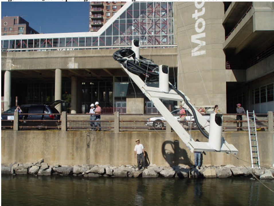
Figure 15. RITE Transducer Mount Deployment
