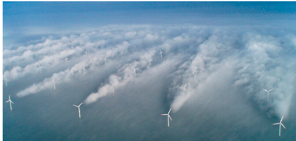
Figure 17. Wake effects from Vattenfall turbine array in the North Sea. Photo via NOAA [63].
